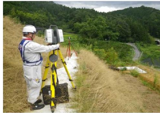
Surveying with a laser scanner
